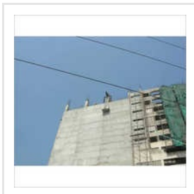
Heavy Structural Work
