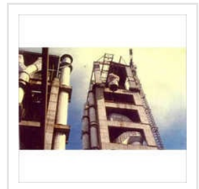
Dismantling And Erection Services
